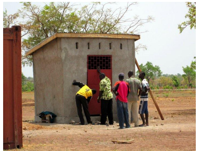
Batteries rest in this building built by Bernie and friends.
